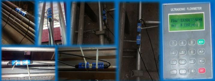
Thermal Power Plant Hydraulic Fluid Flow Study: Support in management of Chemicals & Coolants through flow measurement | Temporary measurement at 96 points within a span of 72 hours | Measurement medium – Phosphate Ester (Turbine Coolant / Fire-resistant oil) | Pipe sizes - 15 to 25 mm
