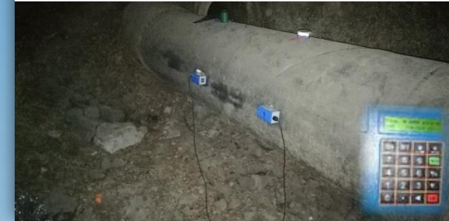
650mm, WTP Inlet Mild Steel Pipe
