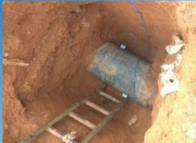
900mm, Raw Water Pumping Station Outlet Mild Steel Pipe
