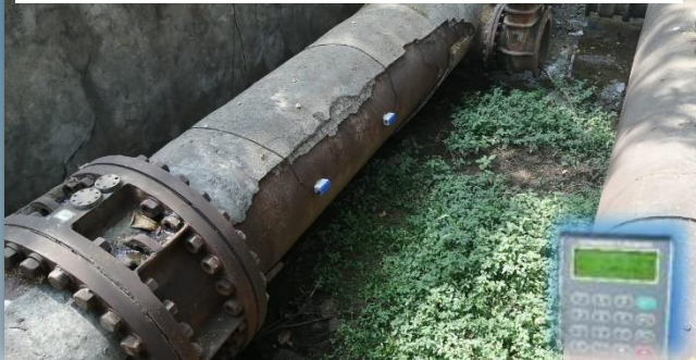
900mm, Raw Water Pumping Station Outlet Mild Steel Pipe
