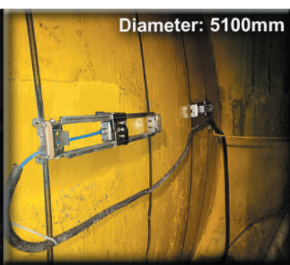
Penstock Monitoring - Clamp-on Sensors
