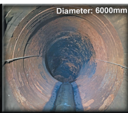
Penstock Monitoring - Inside Pipe Wedge Sensors
